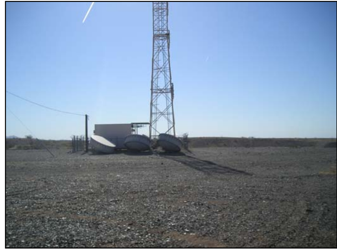
Photograph 6: View from Vidal Junction candidate location, facing east.
